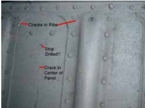
Figure 1. Cracks on Secondary Aircraft Structure
