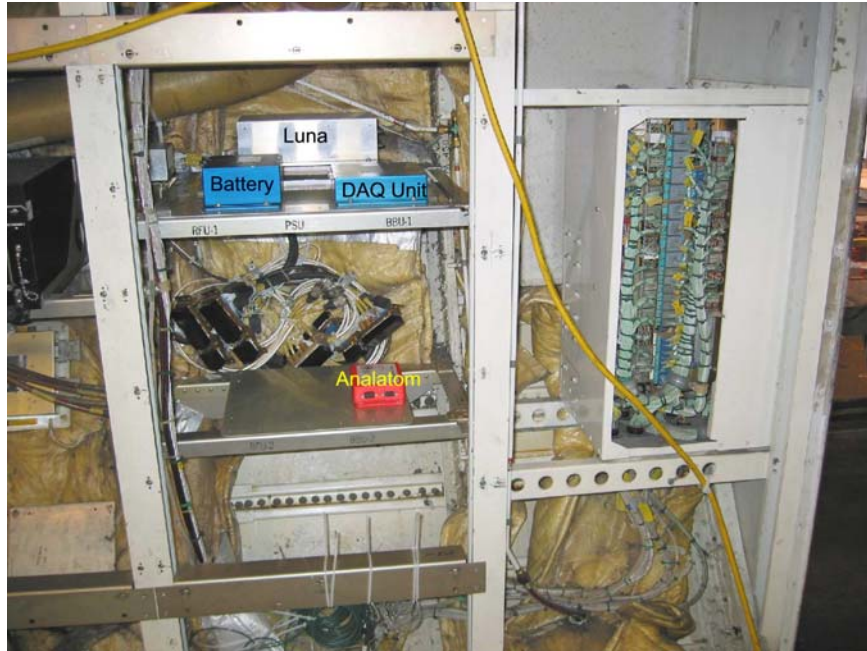
Figure 3. Boxes installed inside cargo wall.
